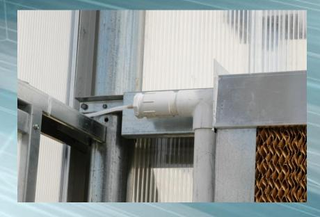
Tube drains outside into gravel basin or into floor drain
